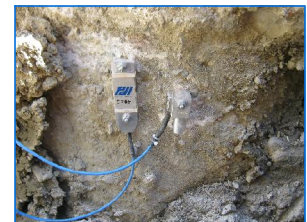
STRAIN-GAUGE E ACCELEROMETRO
